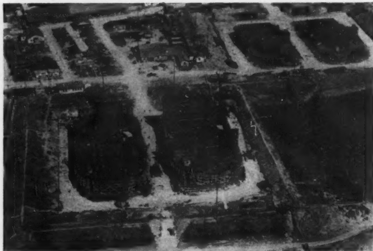
Sections of floating drydocks were built in basins, partly above tide level and "locked-out" by filling the basins with water. (ENR March 22, 1945, vol. p. 390.)
